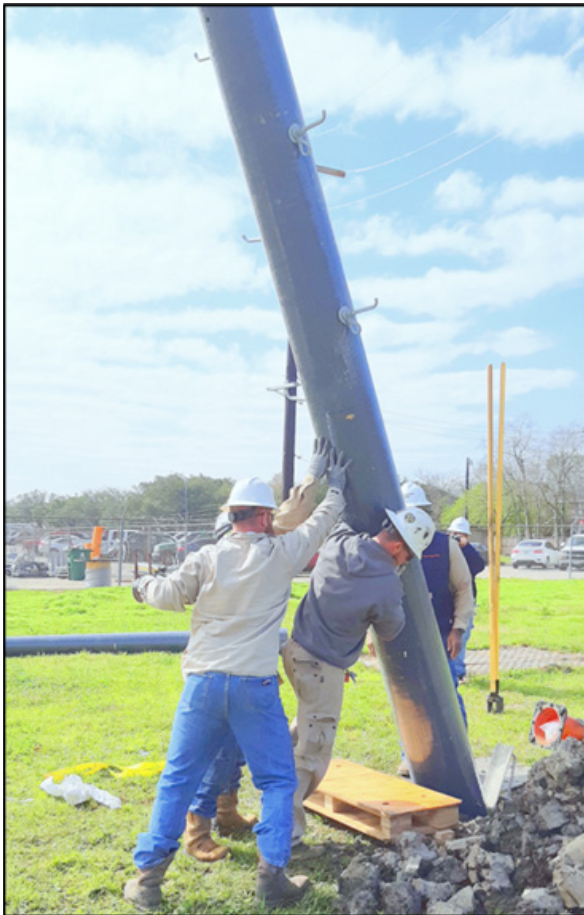
Figures 8a/8b: (a) Setting the base module with steps pre-installed. (b) Rotating the base for proper alignment.
