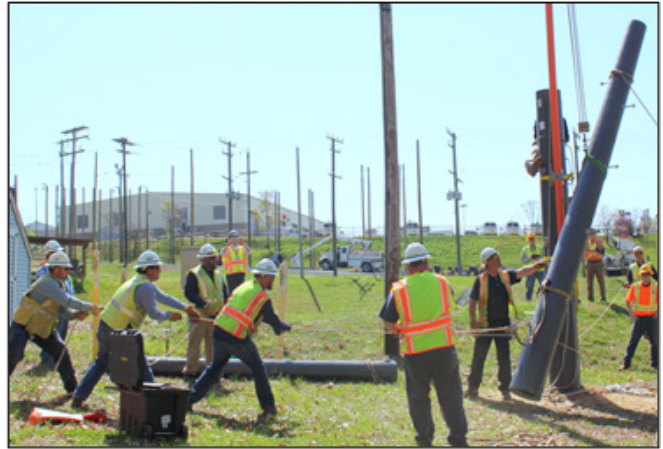
Figure 21: Three workers pull hand over hand, raising the module, while listening for directions from the observer.
