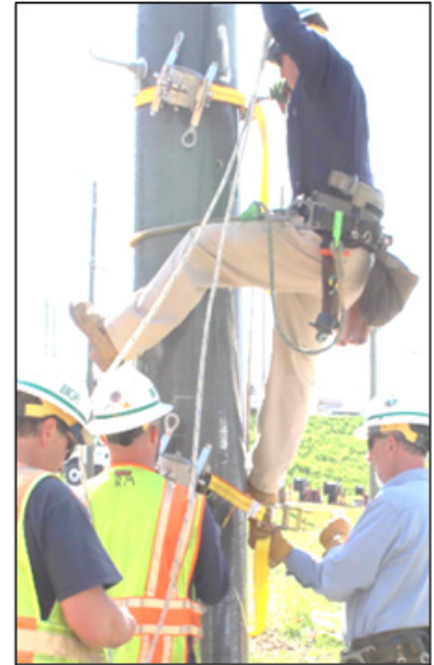
Figure 12: Installing a clamp assembly in preparation for mounting the gin pole.
