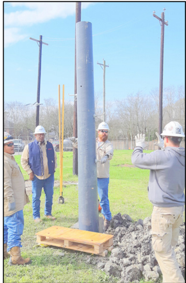
Figures 8a/8b: (a) Setting the base module with steps pre-installed. (b) Rotating the base for proper alignment.
