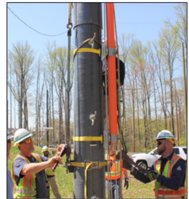
Figure 24: Compressing the joint from the ground using 2 ton lever hoists.
