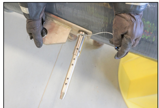
Figure 18: Rotating the retention pin to find the most suitable hole to keep the plate tight against the module wall.
