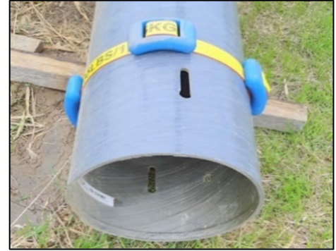
Figure 20: Adding ballast weight to the base (required for RSM-04 module only).
