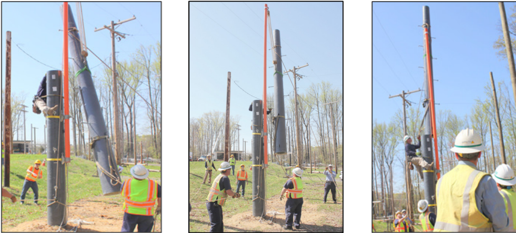
Figure 22: Crew lead is observing and directing the crew as the module is raised with a smooth consistent pull until the base has cleared the upper edge of the bottom module ( far right ).
