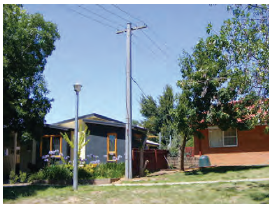
One of the 28,000 composite poles to be installed as part of the upgrade.
