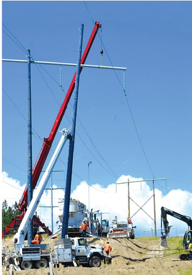
*Composite poles find most application in cases where existing structures are not lasting as long as expected due to attack by wildlife, environmental conditions or pollution.*
