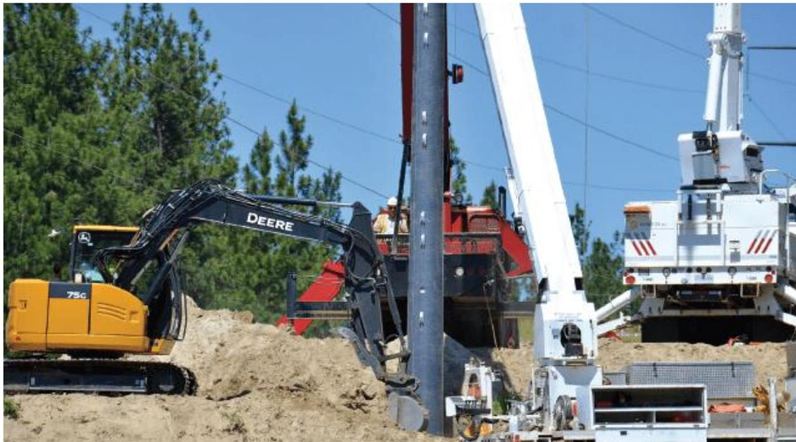
*Assembly of modules that make up composite poles must be done correctly or there is risk of slip joint compression in service.*
