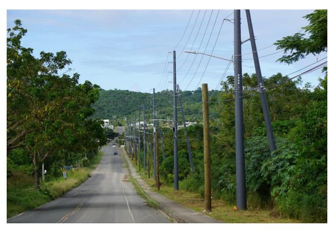
A line of RS FRP composite utility poles installed in the U.S. Virgin Islands as part of a FEMA hazard mitigation project. These structures are designed to withstand 200mph (320km/h) wind speeds so as to increase system resiliency and harden the electrical grid from the damaging effects of future hurricanes.
