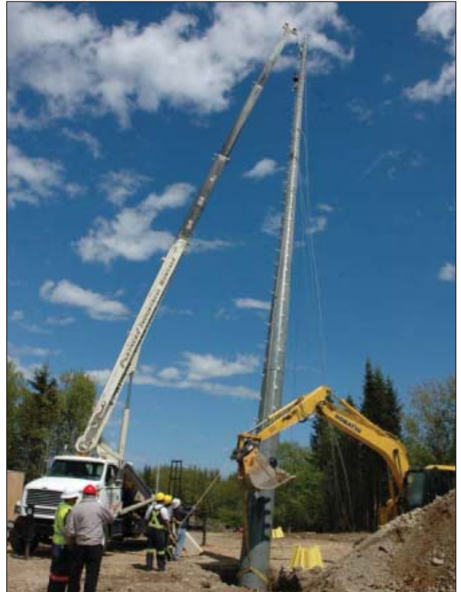
This May 2009 composite RS monopole installation in Nova Scotia provides an example of fast, direct-bury installations. These poles saved thousands of dollars by not requiring foundation materials and by speeding installation — only a crane and a backhoe were used.
