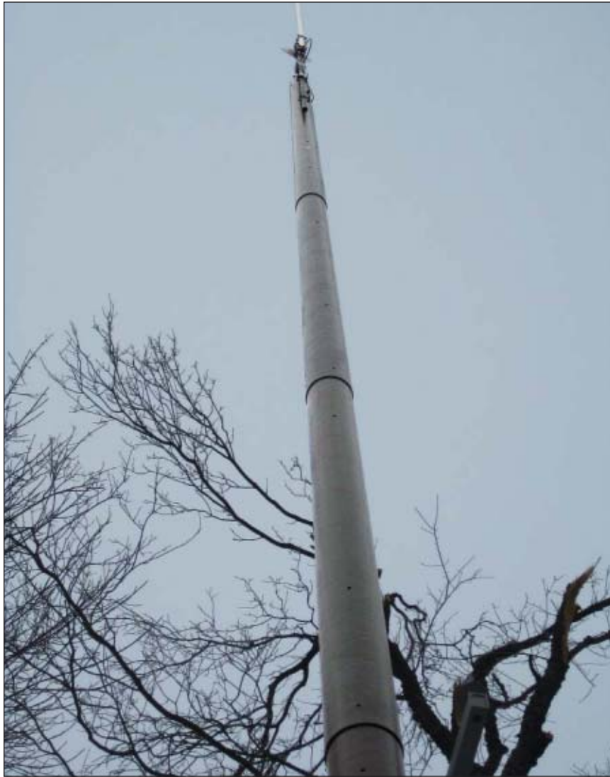
Monopole sections ship in 15-foot modules. The modular construction allows the poles to be easily extended after the initial installation if a change in pole use makes such a change desirable.
