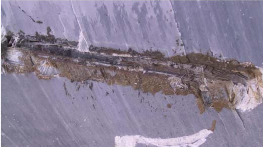
**Figure 9:** Structural damage, module replacement may be required.
