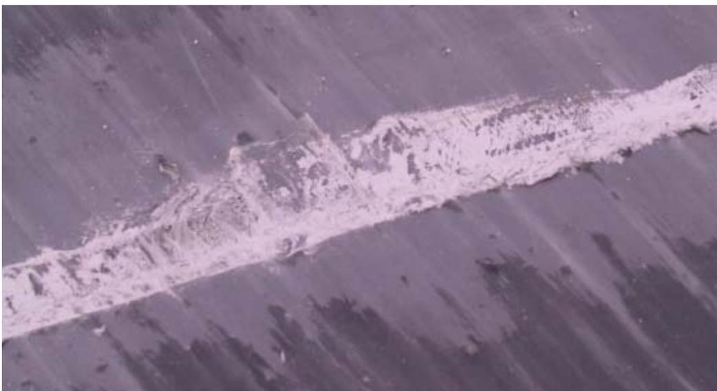
**Figure 8:** Surface gouge damage, maintenance required.
